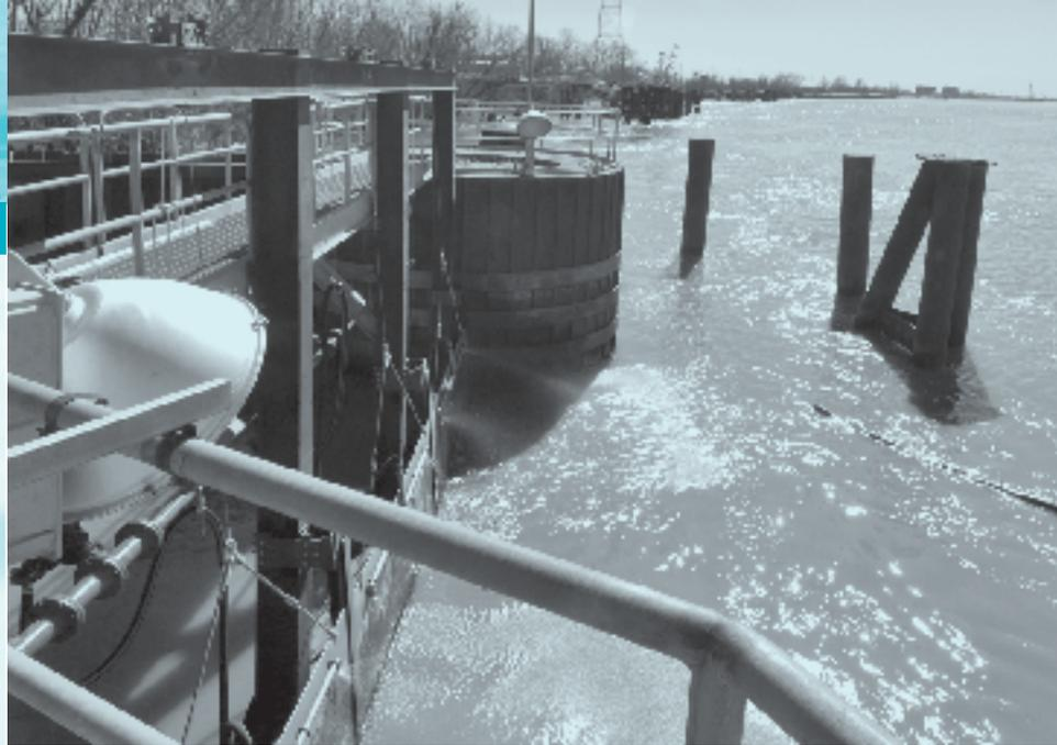
New Orleans' only source of potable water is the Mighty Mississippi River. Raw water is brought into two treatment plants by four intakes like the one shown here. The intakes are protected from ships and barges by concrete barriers and wooden pilings. The water is then treated via a complex purification process at the Carrollton Water Purification Plant for East Bank customers and at the Algiers Water Treatment Plant for West Bank customers.
