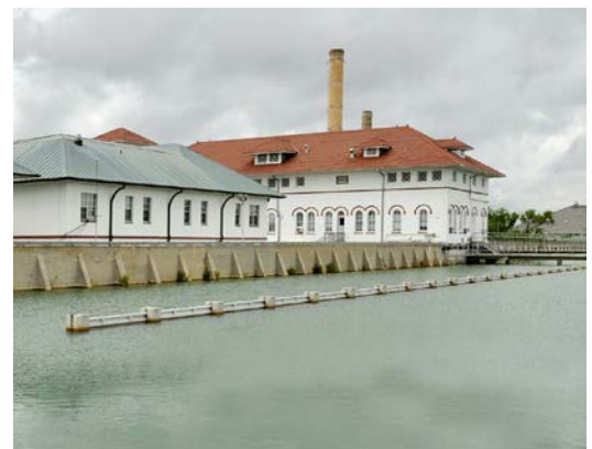
Carrollton Water Purification Plant
