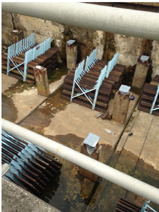
L3 Sedimentation Basin Flocculator Rehab
