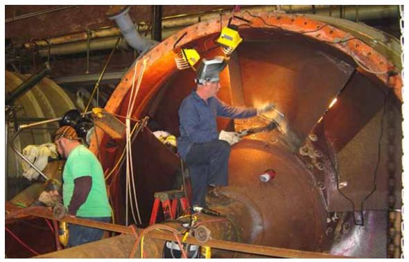
When one of the pumps at Drainage Pumping Station No. 3 began to "chatter" and make a loud noise, it was discovered that 5 of the 8 impeller blades were cracked. The Board's own employees from Facility Maintenance disassembled the pump, gouged out the cracked areas and weld-repaired the blades.
