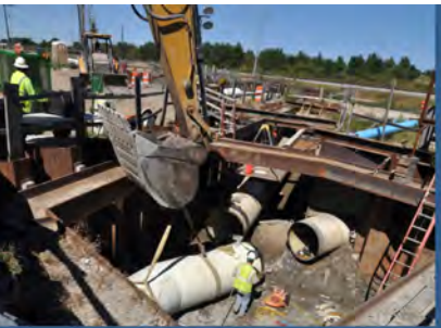
(left) This photo shows crews replacing a 48" waterline in the construction of the Florida Avenue Canal Project, a part of the relocation and replacement of waterlines included in the Southeast Louisiana Urban Flood Control Program (SELA). Besides waterline replacement being a part of SELA, the city has a larger city-wide multi-year infrastructure repair/recovery waterline replacement program funded by FEMA. This program is designed to restore the city's water distribution system. To ensure that the city is maximizing available funding, various agencies are involved in the co-ordination efforts of the program.
