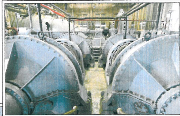
Drainage Pumping Station No. 5, located on the east side of the Industrial Canal at Florida Avenue, was inundated with flood waters in 2005. It is back in operation after much hard work and dedication to refurbish and repair the pumps, electrical systems and buildings.
