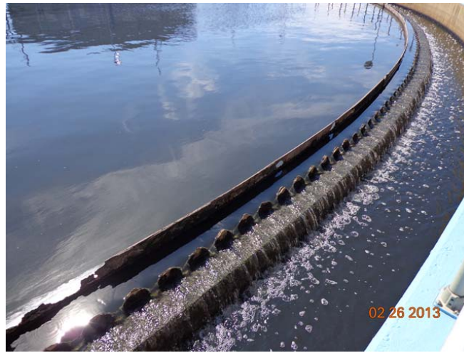
Figure 3 Primary Clarifier Weirs to be Refurbished in 2013
