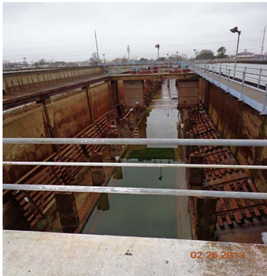
G4 Sedimentation Basin under Repair
